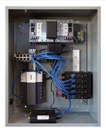
Wattstopper POWER SUPPLY for JACE 8000 / 24VDC 1.0 AMPS Part No. NB-PS1
