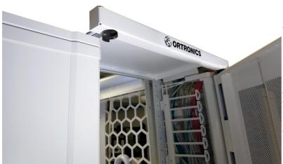
The Mighty Mo 20 Heavy Duty Security Door offers a lockable, dual hinged door, designed to secure open racks in data rooms and colocation facilities. The Mighty Mo 20 open frame rack easily adapts with upper and lower door supports to provide for a conversion of a single rack or an entire row of racks. The doors assist in making the Mighty Mo 20 even MORE data center ready by enclosing the electronics as well as protecting and securing data connections.
